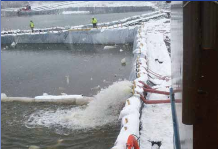
4 lines opened for flood control.
