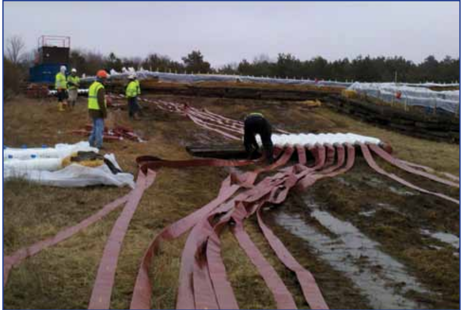
Floc Hogs installed with 100' of hose between banks.
