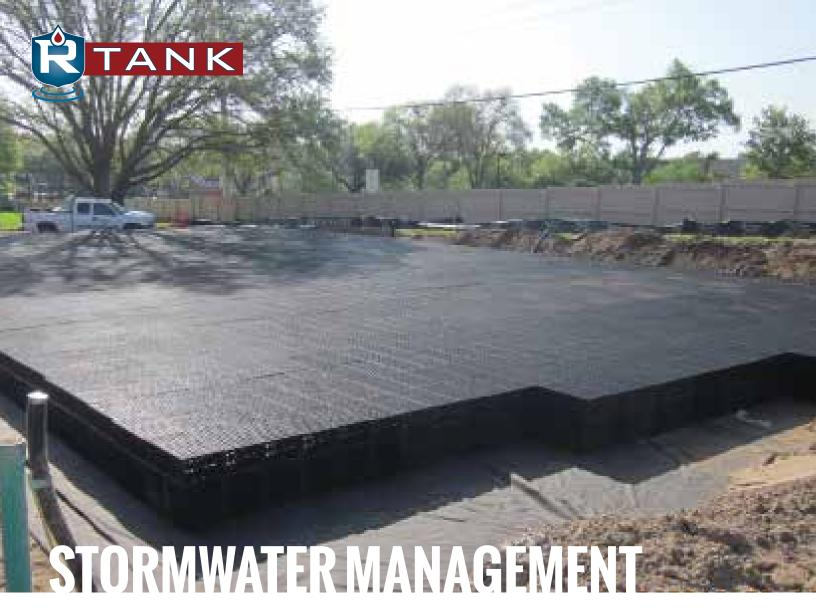
R-Tank stormwater systems provide underground storage of stormwater. After a rain event fills the R-Tank, stormwater can flow into the drainage system, infiltrate into the ground, or be reused. The system is an alternative to stormwater basins and a more efficient, space saving alternative to other underground systems for detention, infiltration, and recycling stormwater.
