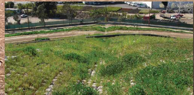
60' wide letdown 4 years after installation.
