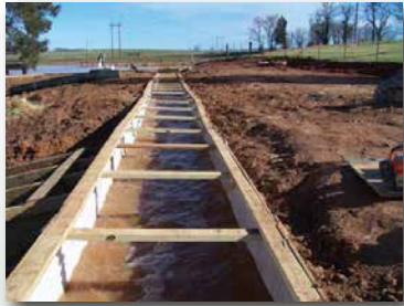
Gravity Flow to Flume
