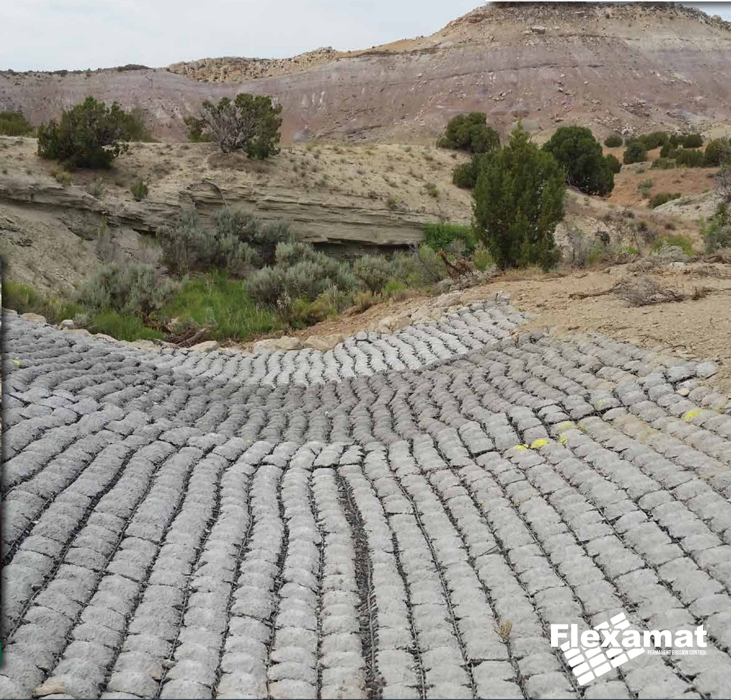
Exposed high pressure gas pipeline.
