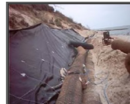
Helical Anchor Tie Back
