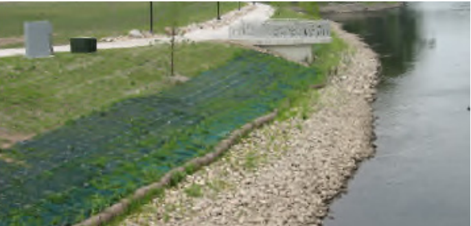
System Solution of TRM, Coir Log & Riprap
