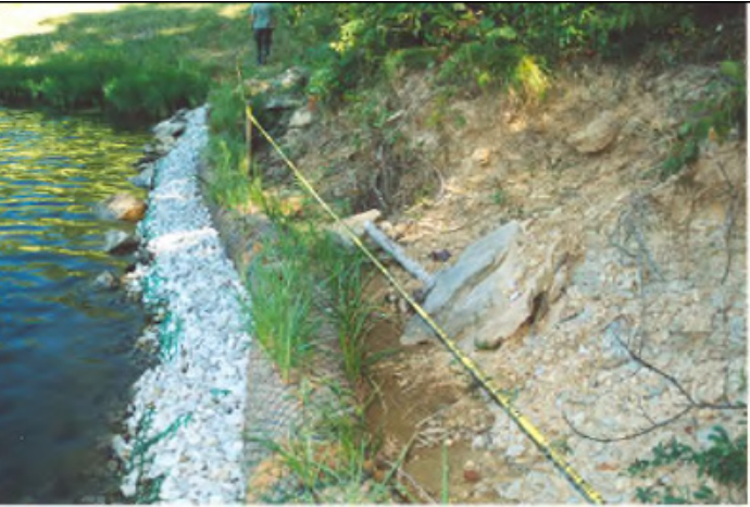
Shore Line Protection at Lake Lemon, Indiana (One Month Old) 16” Vegetated Coir Log with Rock Roll Chambered Revetment
