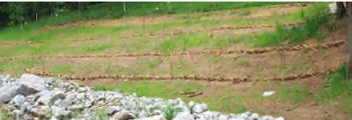
Example of Slope Contouring
