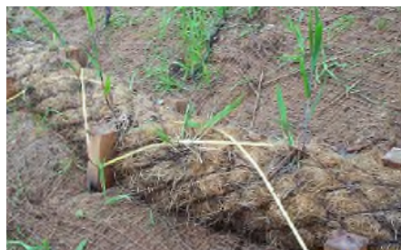
Coir Logs with Standard Staking & Lacing
