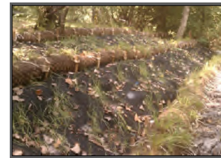
Coir Log Tied to Revetment Structure
