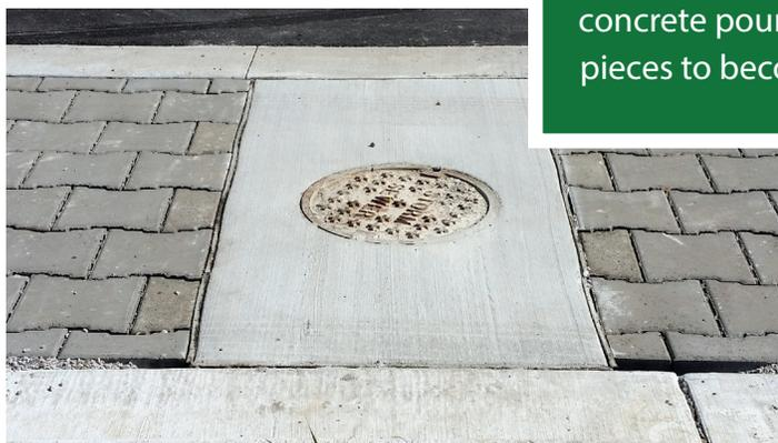
PaveDrain blocks work with existing infrastructure and can be used as the form for small concrete pours. No small, cut pieces to become dislodged.
